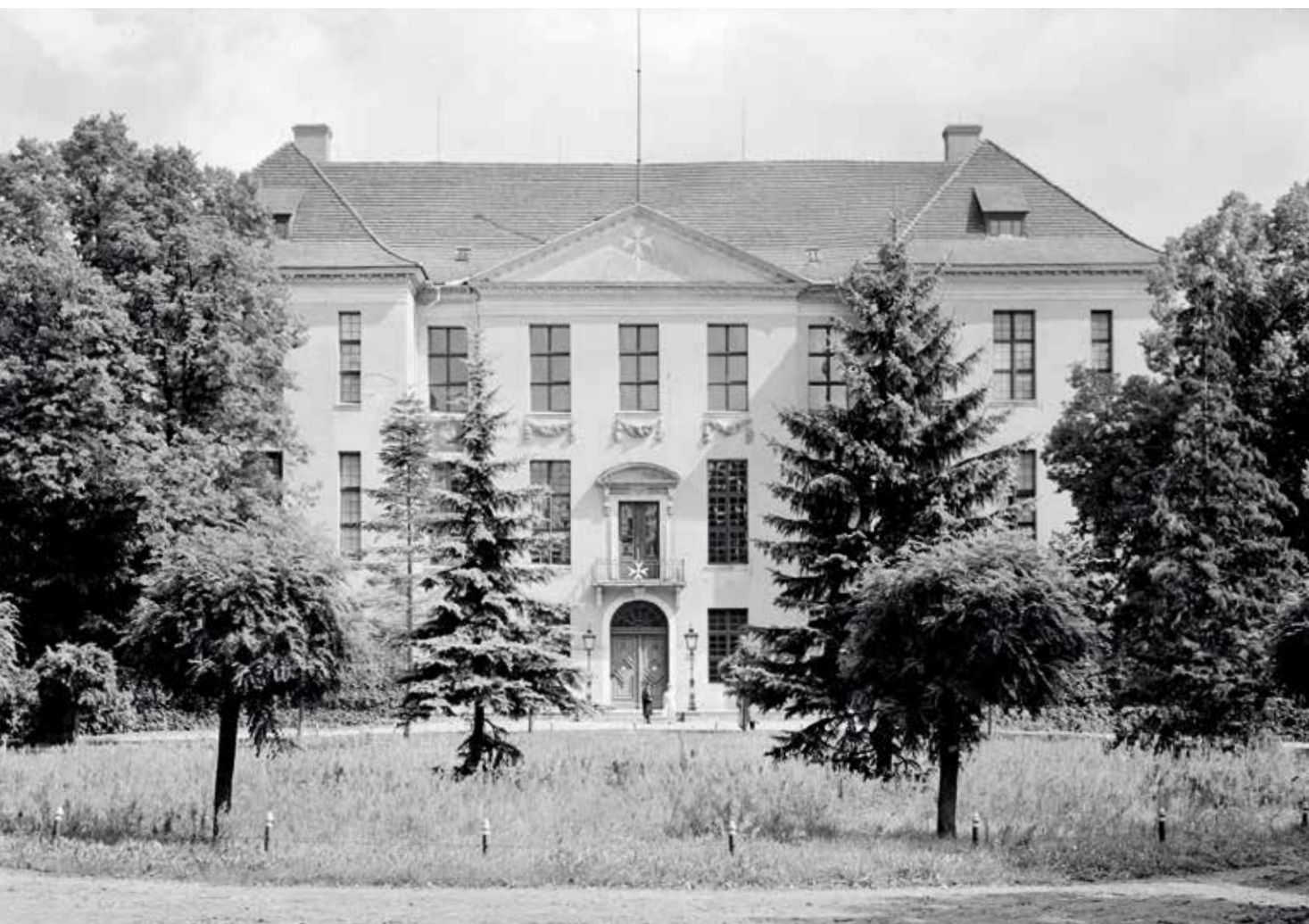
2. Sonnenburg facade before 1940; it was rebuilt from 1662 to 1667 by order of Johan Maurits van Nassau-Siegen (Bildarchiv Foto Marburg)
