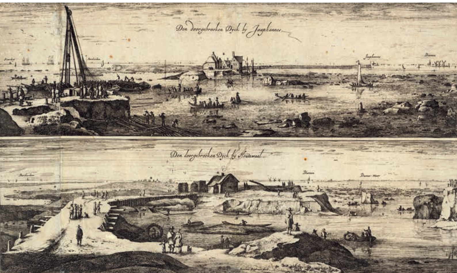
3. Roelant Roghman, Breach of the Diemerdijk, 1651 . Visible in the foreground of the upper picture is a pile frame used to insert piles for a new part of the dike. In the picture below, the dike repair has already been partially completed (Amsterdam City Archives)
