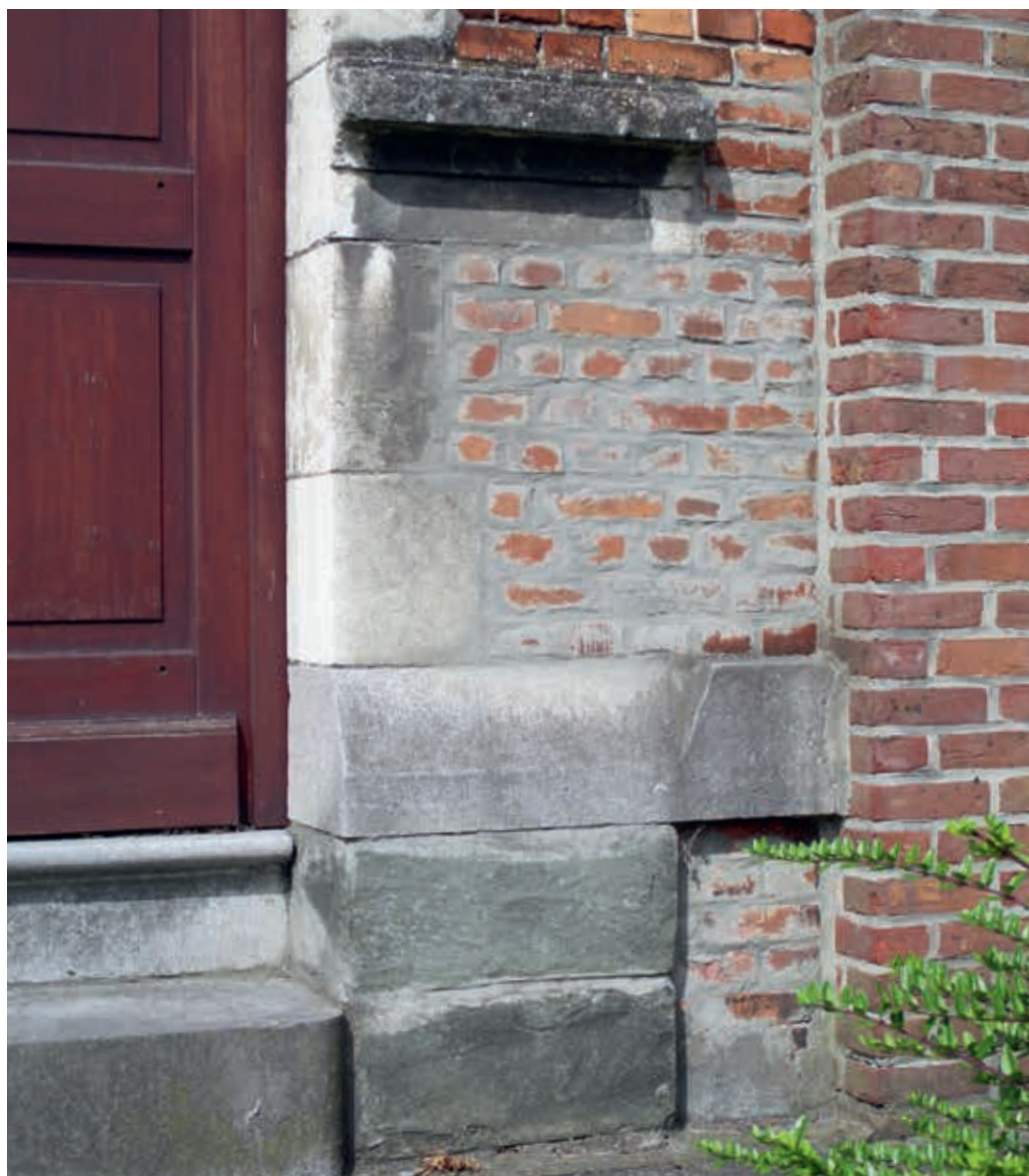
12. The specific splitting contours in the stone in various places in the Sint-Gerardus school demonstrate the authenticity of the reconstruction of the model school from the Modern Village
