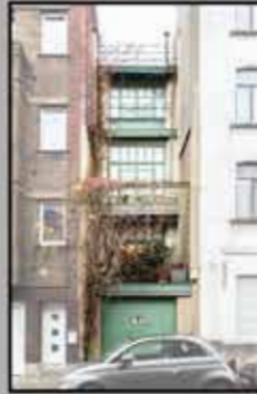
1902 - Calvijnsstraat 5 Personal residence - Rear facade
