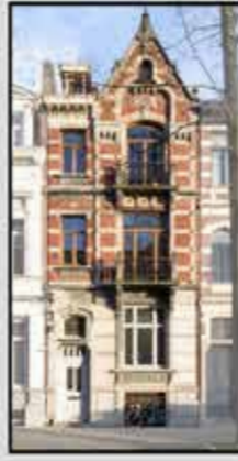
1894 - Brabançonnelaan 7 First personal residence
