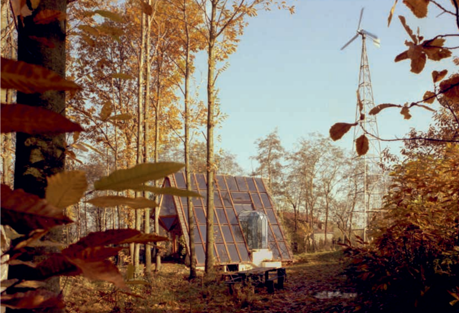
15. South elevation of Luc Schuiten's house (Maison Oréjona) clad with solar panels, with wind turbine in the garden, Overijse, 1977 (photo Luc Schuiten, c. 1980)
