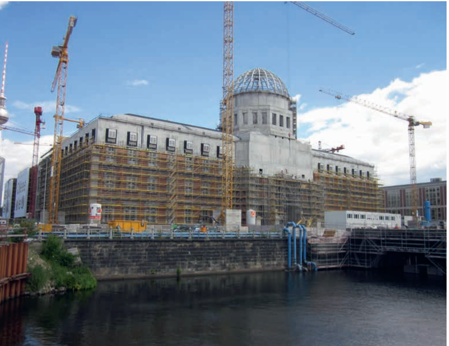
3. The Berlin Stadtschloss (City Palace) under (re)construction, July 2016 (author's photo)
