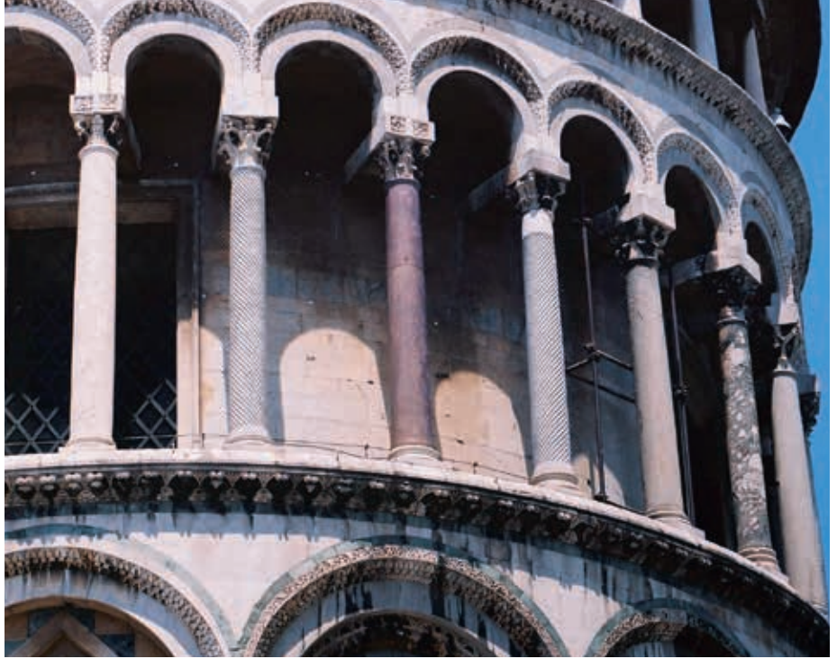
2. Pisa Cathedral, spolia columns in the dwarf gallery of the apse (author's photograph)
