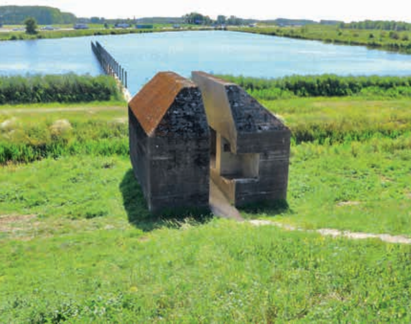
3. A layer added to the history of the place. This divided bunker, once known as Bunker 599, offers visitors to the Diefdijk Line a different perspective of the surroundings. A joint project of RAAAF and Atelier de Lyon, 2013 (author's photograph)
