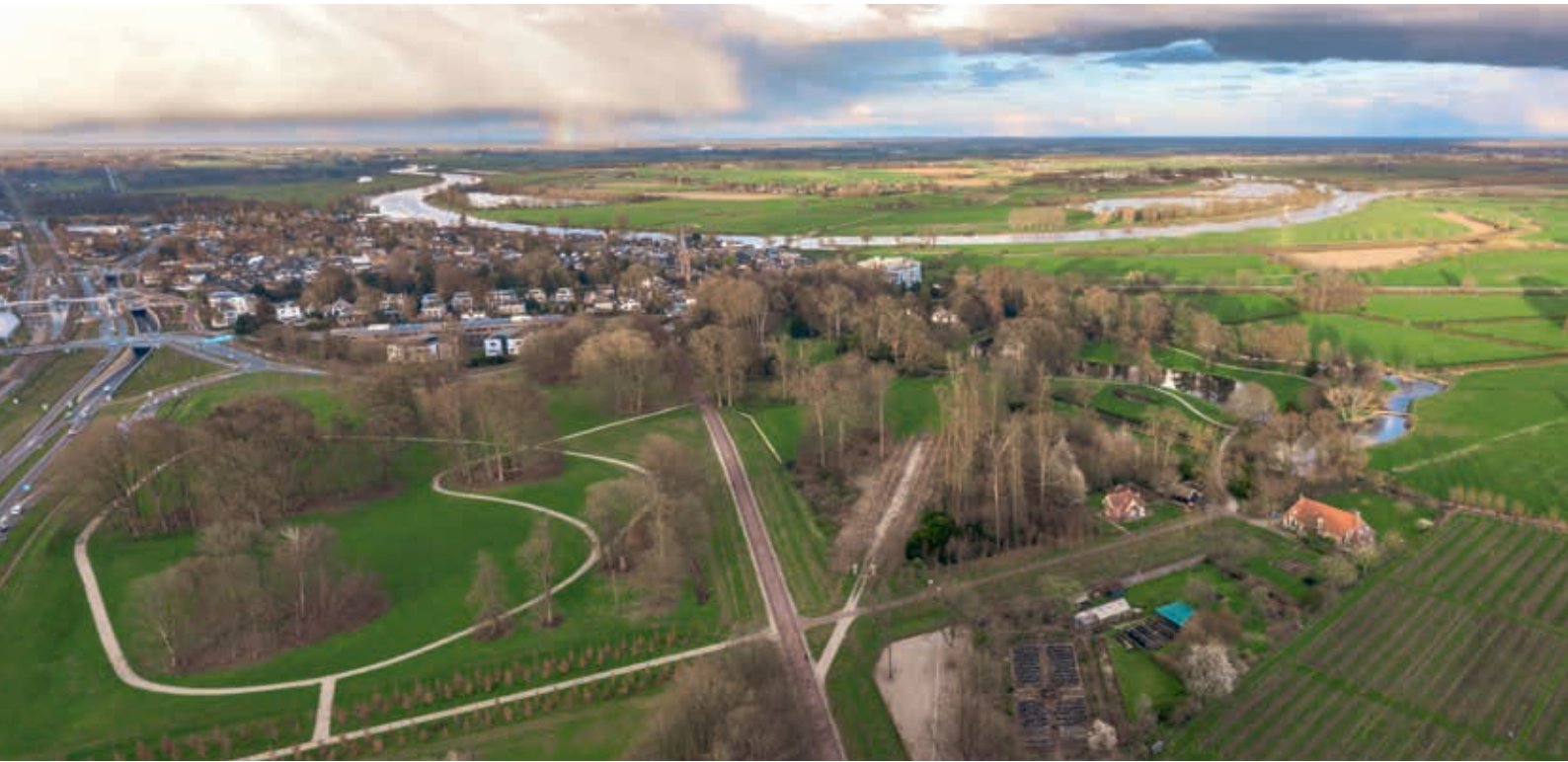
10. The reconstruction of the provincial highway provided the opportunity to enhance the designed landscape in the heart of the Hof te Dieren estate in the municipality of Rheden (photo MVO TV)
