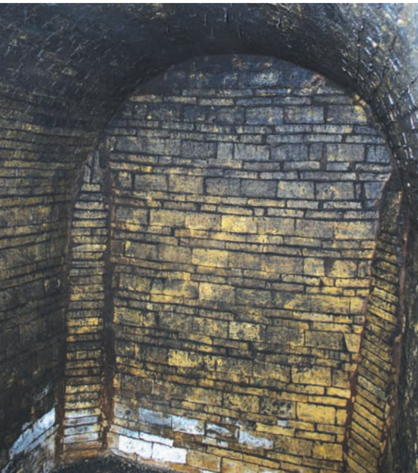
11. Structure of the interior of the excavated rainwater cistern on Lamme van Dieseplein (M. van der Wal 2015, 15)
