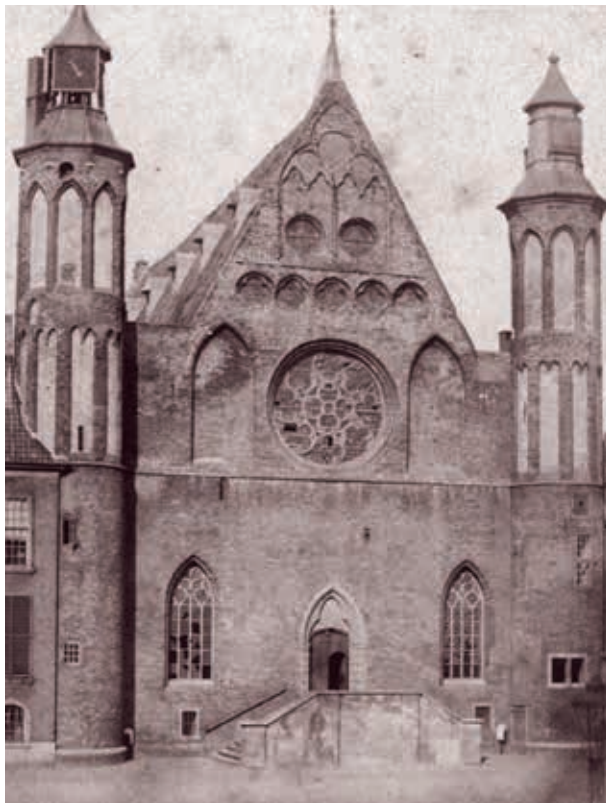
3A. The west front of the Great Hall in 1860, showing the tracery of lead-covered wood inserted in the two pointed-arch windows in 1814, and the rose window. The gable displays the original steep wall line that is aligned with the original roof construction. Only the gable shoulders have been raised (The Hague City Archives)
