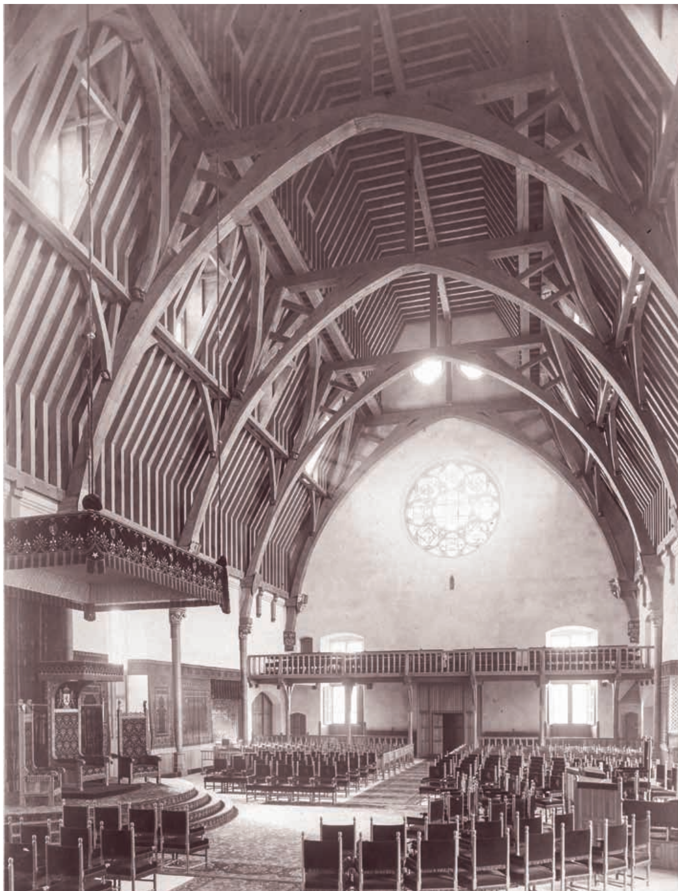
10. Interior of the Knights' Hall after the restoration with reconstructed timber roof, 1905 (Cultural Heritage Agency)
