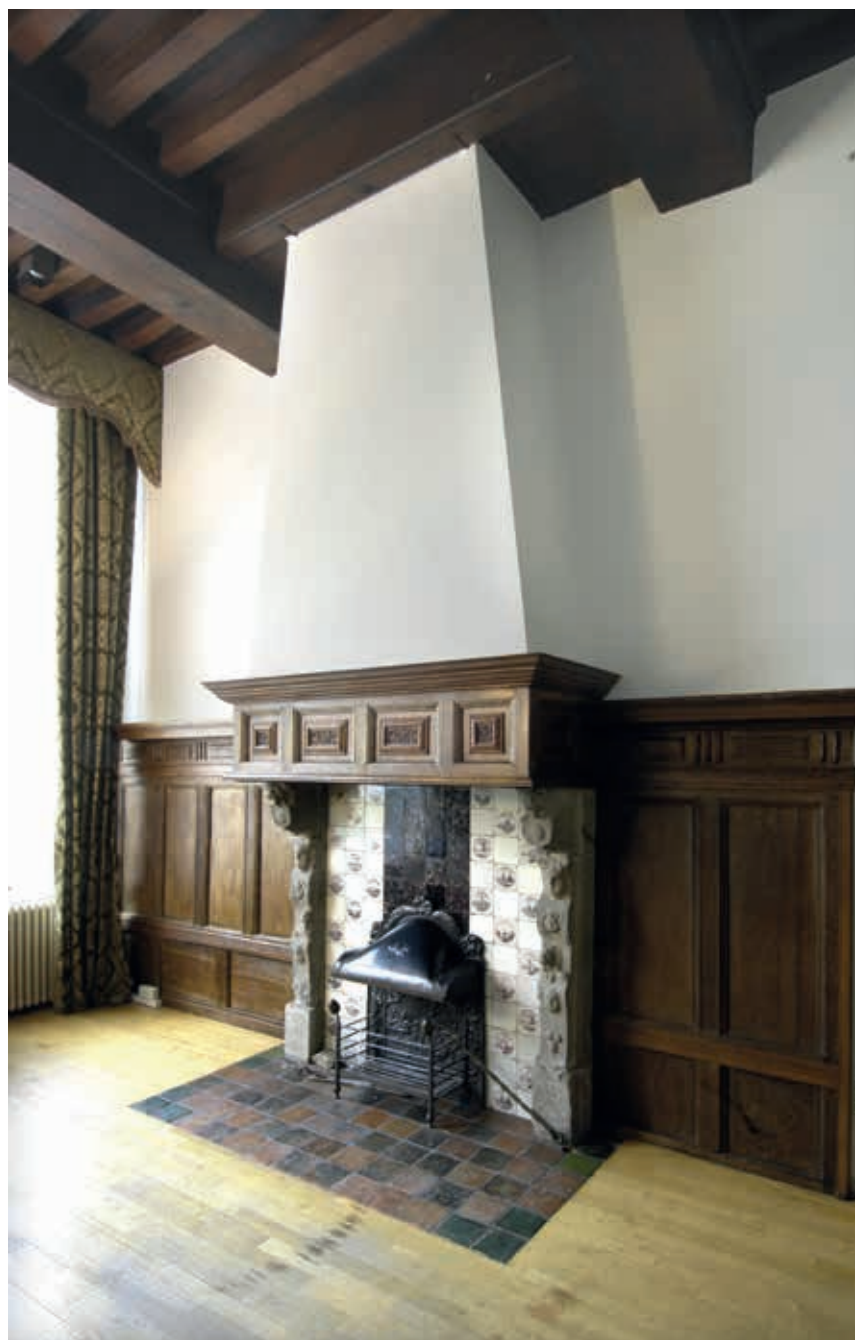
7. Head-height panelling of wainscot was used in houses and other buildings well into the seventeenth century. Example of reused panelling in Keizersgracht 123 in Amsterdam (photo Han van Gool, Monumenten en Archeologie, Amsterdam)
