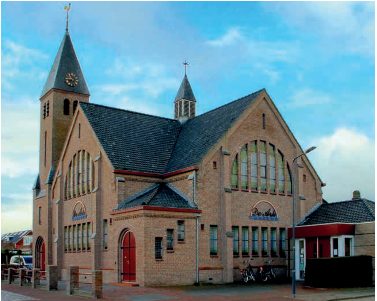
12. P.S. Dijkstra, Reformed Church on Veerweg in Kamperland, now De Ark (photo Marieke Kuipers, 2022)
