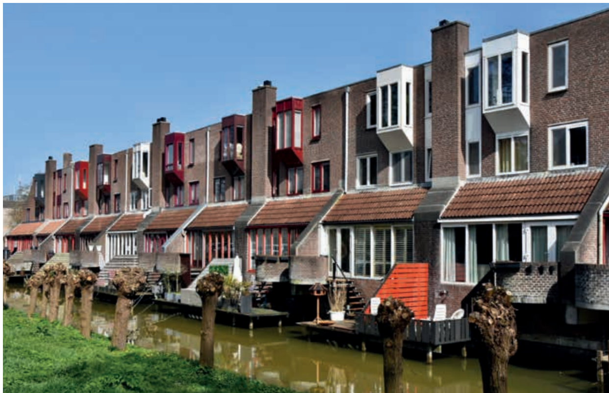
2. Pietro Hammel, water dwellings in the Doorslag district of Nieuwegein (photo Daphne Luijters)
