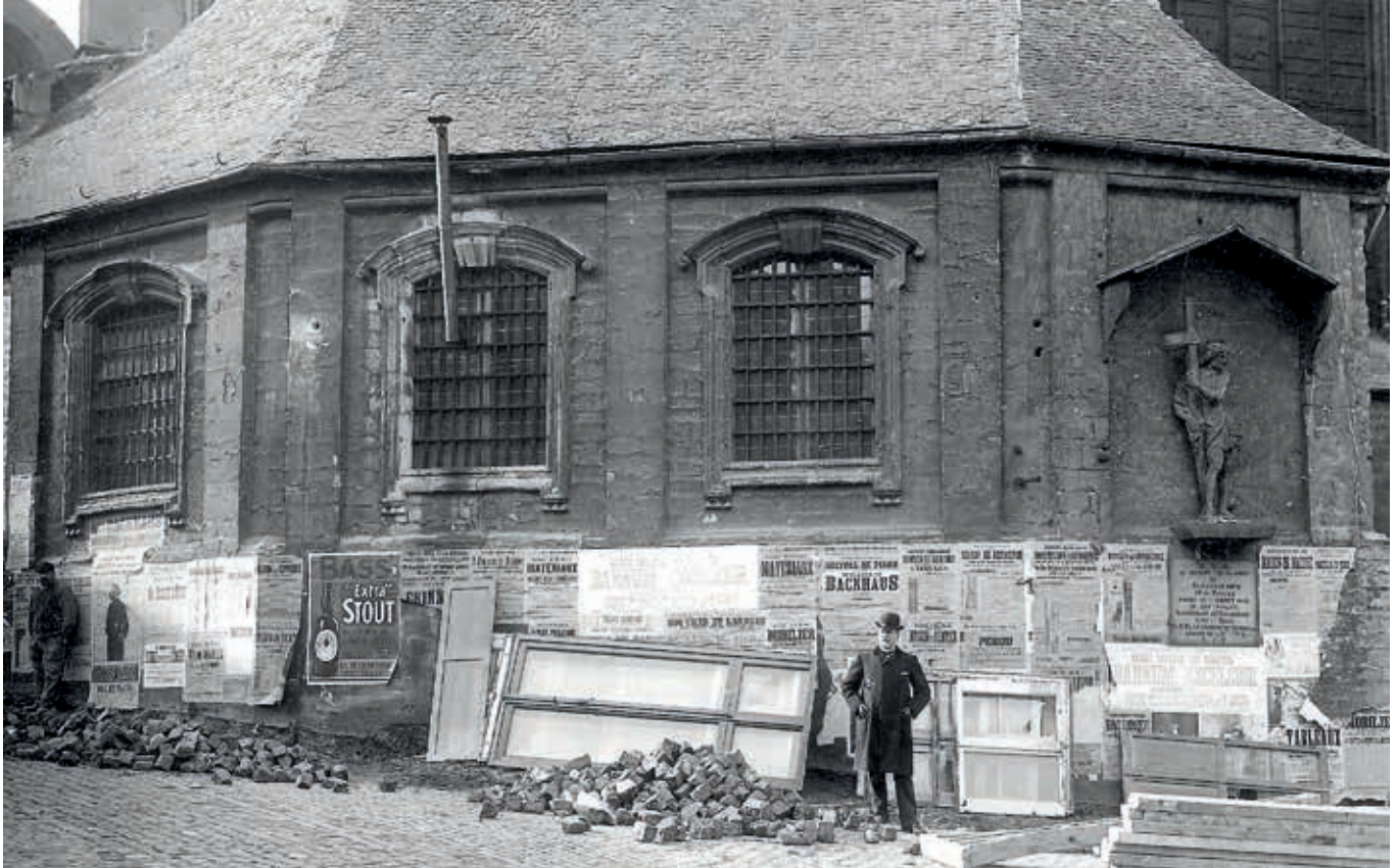
7. Demolition materials are visible in the photographs taken during demolition works in Brussels between 1860 and 1940. This photo, taken in 1907, shows sorted timber beams, bricks and demounted windows (photo Comité d'Etudes du Vieux Bruxelles, KIK-IRPA, Brussels)
