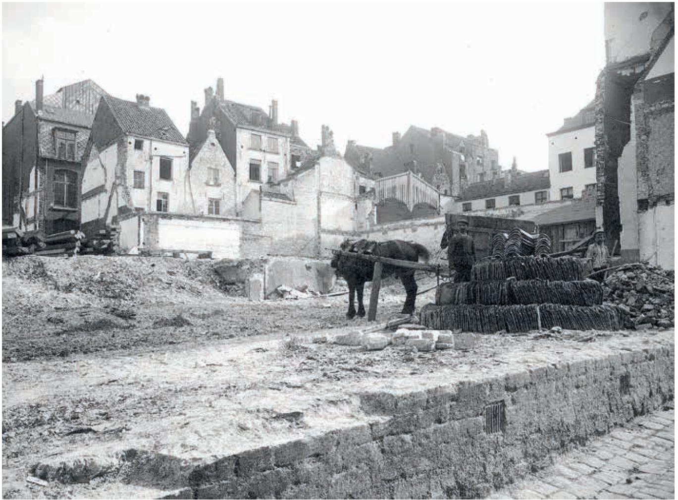
9. Sorted roof tiles and timber beams ready for transport in 1911 (photo Comité d'Etudes du Vieux Bruxelles, KIK-IRPA, Brussels)
