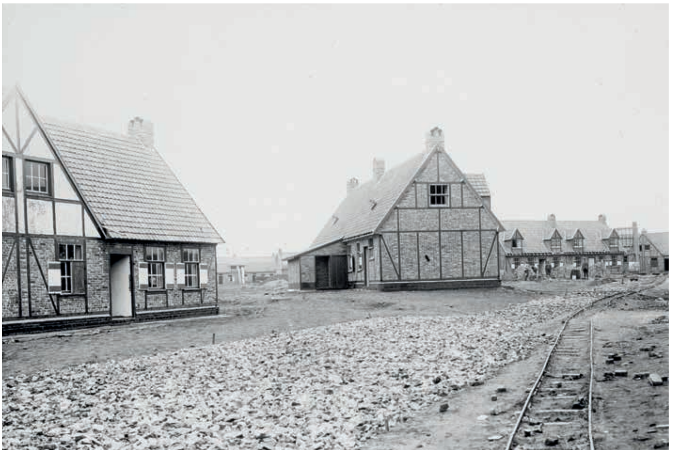
8 AND 9. Semi-permanent dwellings under construction in Ligywijk, Ypres in October 1921 (KU Leuven, Verwilghen Collection)
