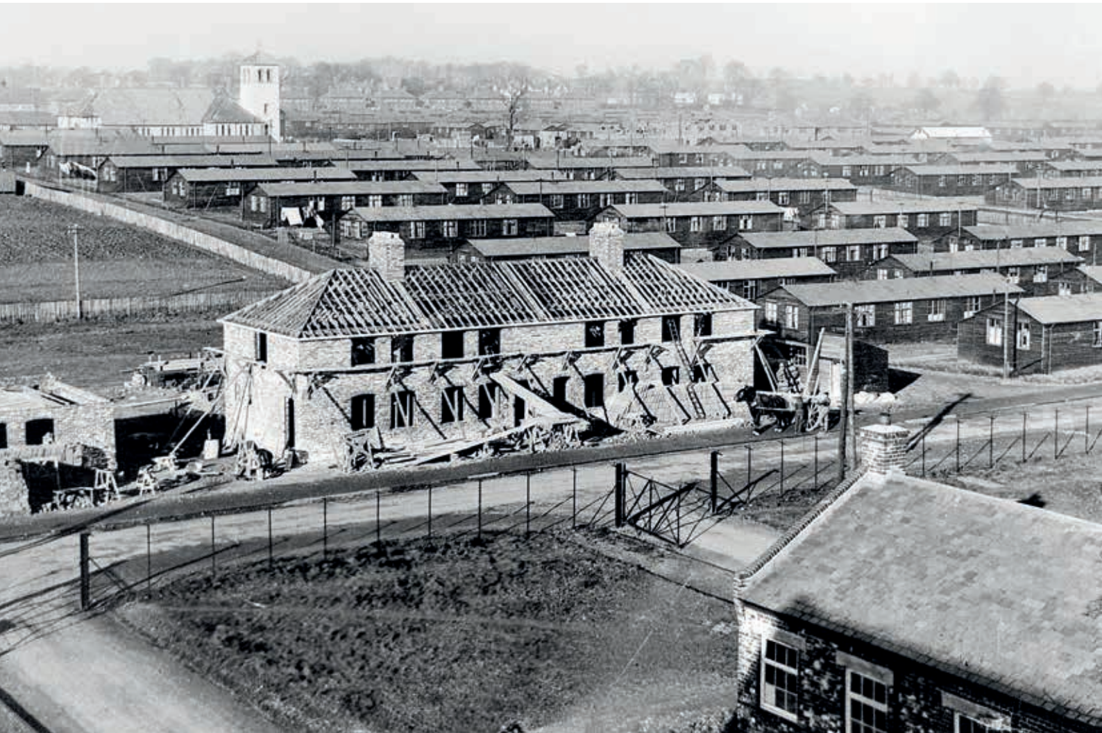
5. Construction of permanent housing shells at Gretna, next to temporary wooden barracks for workers (UK National Archives MUN 5/159/1122/7/19)
