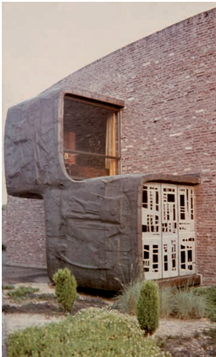
2. The projecting entrance to Huis Witters, clad with copper sheeting recovered from dismantled ships (Photo Jan Mees)
