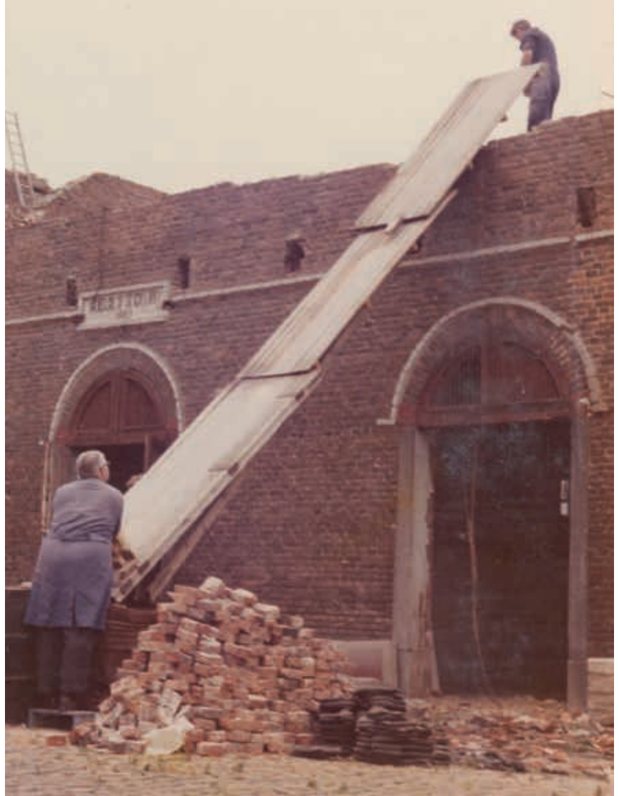
14. Dismantling of the former slaughterhouse in Tienen by the Boncher family to reclaim bricks and roof tiles (Photo Famillie Boncher)
