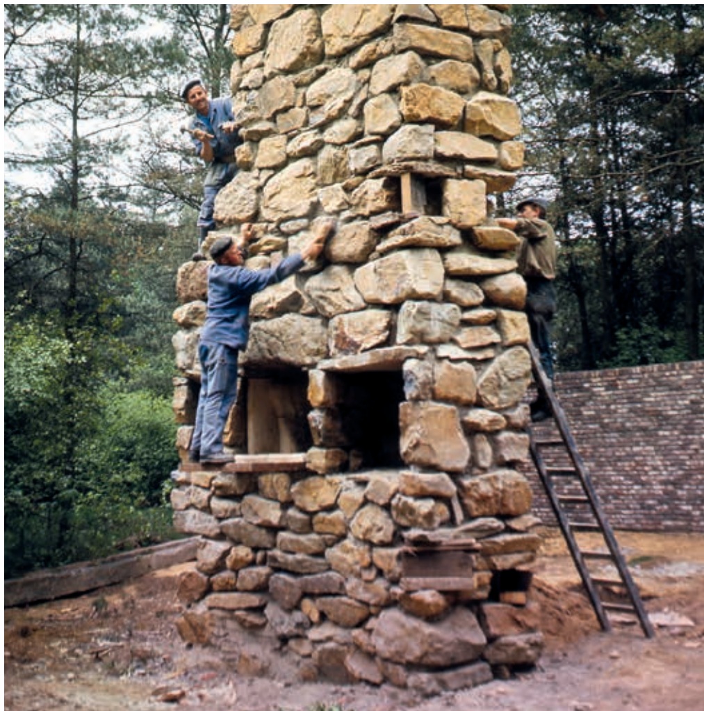
3. The Nijsen House. The central, double-height maaskeien sculpture has just been completed. The rest of the house will be built around it (Photo Familie Nijsen)
