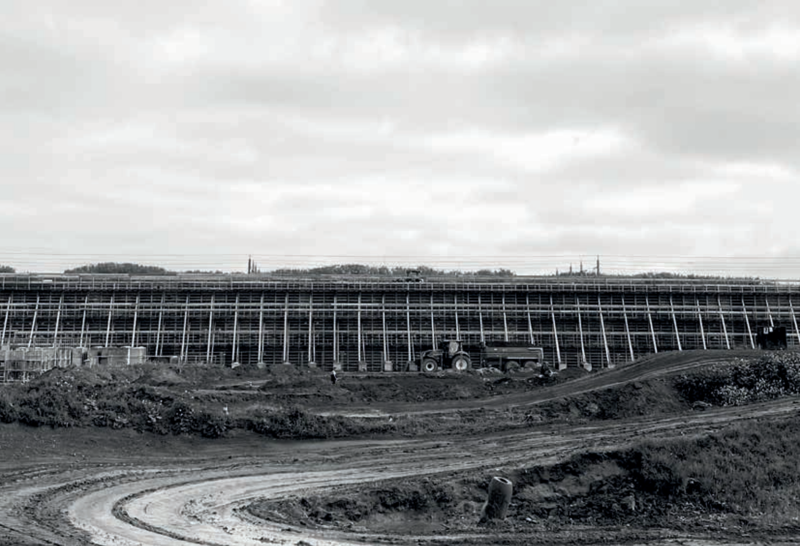
6 AND 7. Construction of an earth wall along the perimeter of a soil bank in Utrecht (photo C. Pradel)
