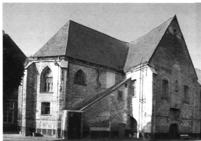
Fig. 8. Church of Maagdendale at Oudenaarde: apse and transept from the north (photo: THOG, May 2004).
