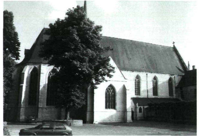
Fig. 12. Church of La Cambre: north side and front of the north chapel (photo: THOC, June 1997).
