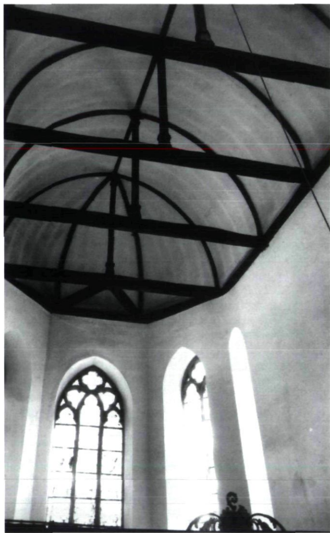
Fig. 15. Church of Soleilmont: choir and wooden barrel vault, fifteenth-century (photo: IRPA-KIK, before the fire of 1963).
