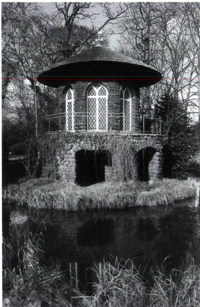
Fig. 27. Park of Vrouwenpark at Rotselaar: early nineteenth-century folly entirely built with material from the ruined medieval church (photo: THOC, February 1997).
