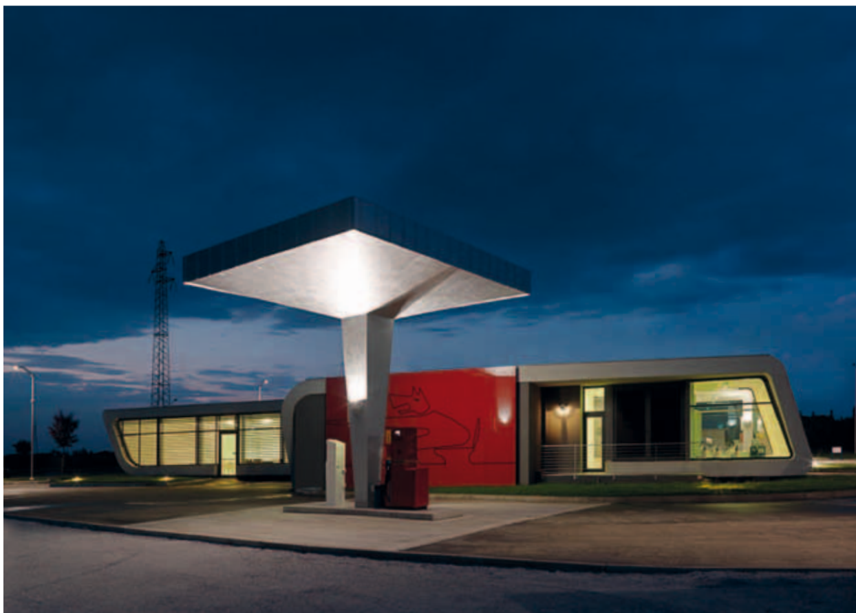
11. Centro Calor benzinstation, Damilano Studio Architects, Cuneo, Italië, 2011 (© Andrea Martiradonna, 2011)
