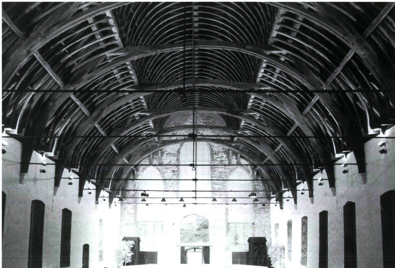
Fig. 24. Hospital of the Bijloke at Ghent: inner view of the great hall to the west and trussed rafter roof of 1251-1255 (photo: THOC, September 1992).
