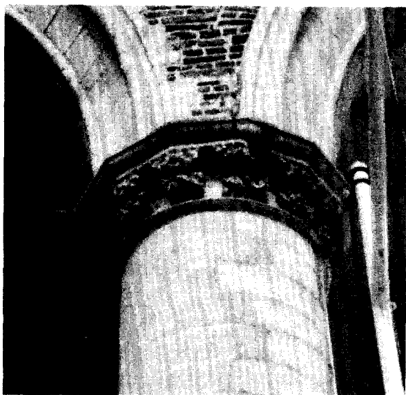
Ill. 3. Second nave capital (ca. 1450) on north side, counting from the west, which was formerly attached to the tower. Notice the quarter section added in 1512, with finer carving (photo author).
