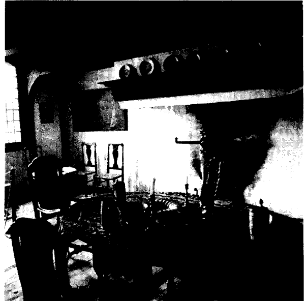
Ill. 13. Interior of the Luykas van Alen House with reconstructed fireplace. Despite New York cold winters and the inefficiency of the open Dutch fireplace, the Dutch continued to build them both in the Netherlands and in America during the 18th century. By that time the English had introduced their smaller, more efficient type (Columbia County Historical Society).
