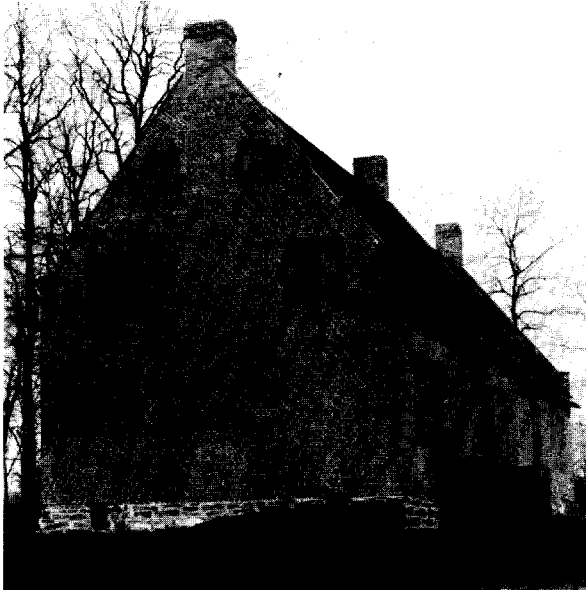
Ill. 12. The Luykas van Alen House, built in 1737. This was a two-room house, shortly after it was built the addition of a hall and room was made. This form of addition, placed on the end of a two-room house, was done with other Dutch houses as well (Columbia County Historical Society).
