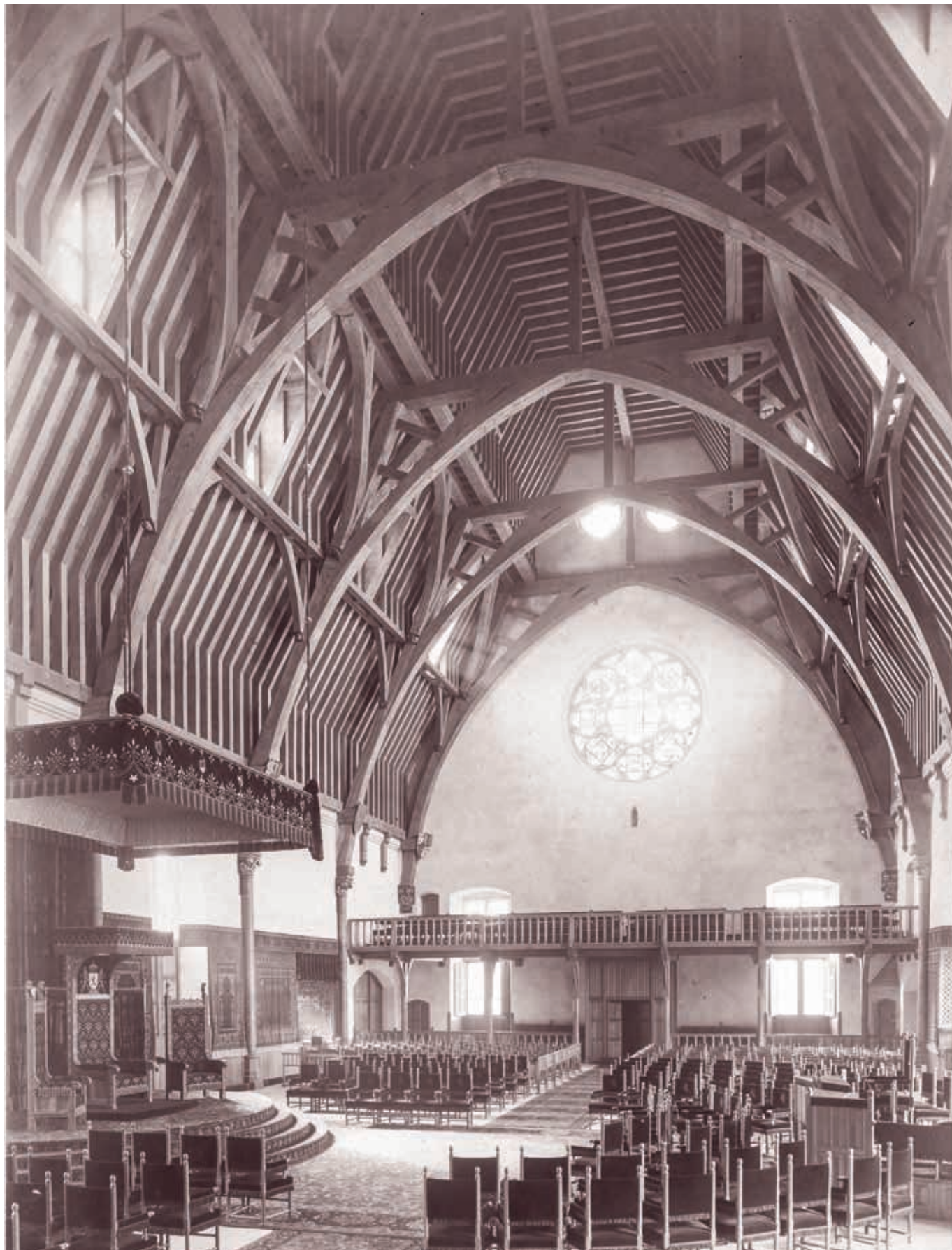
10. Interior of the Knights' Hall after the restoration with reconstructed timber roof, 1905 (Cultural Heritage Agency)
