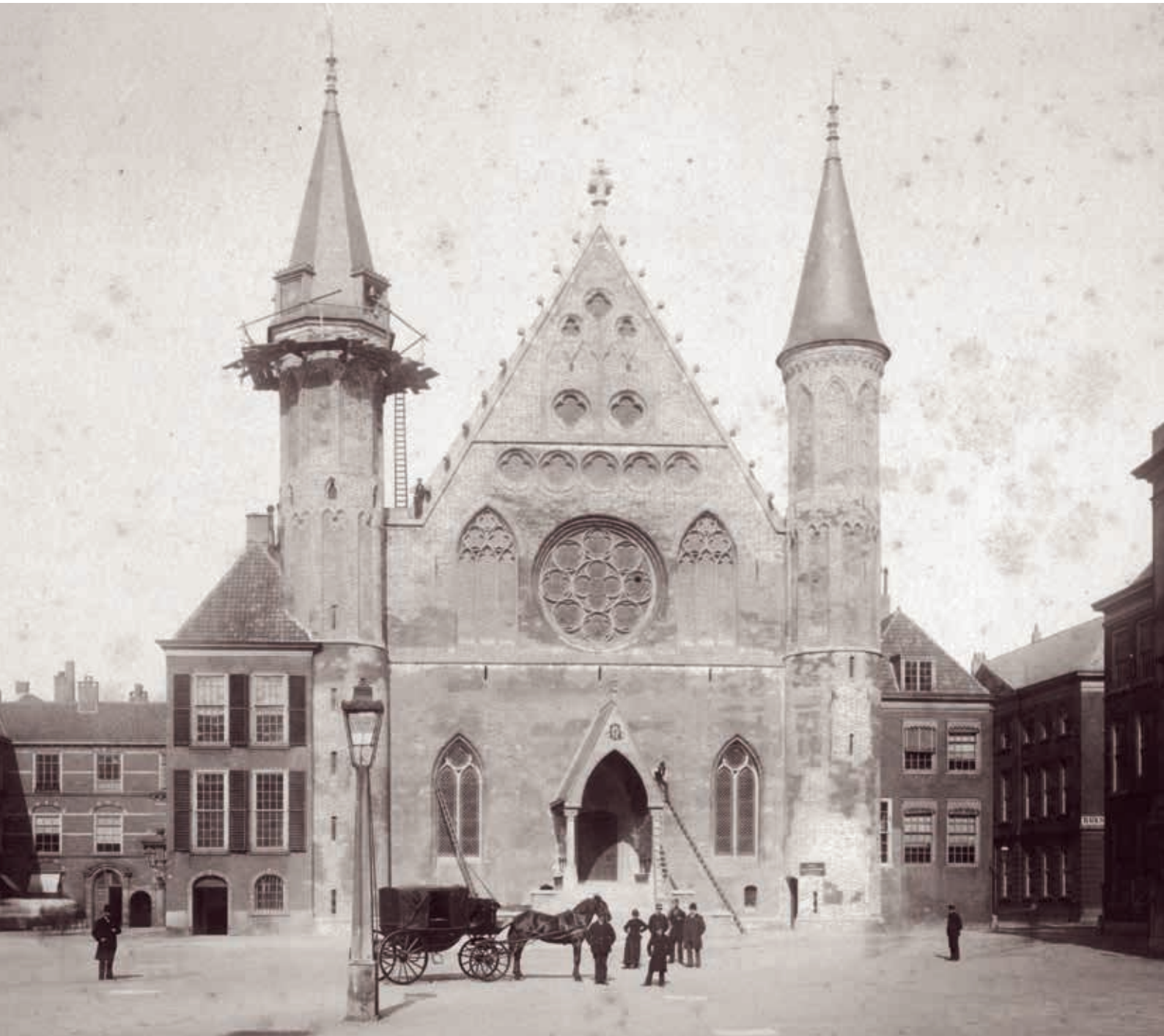
6. The west front of the Knights' Hall during final restoration works in 1880. The reinstated 'medieval' gable emulates the roof line of the 1861 cast iron roof structure. As a result the gable has a larger building mass and the gable wall line a shallower pitch than the original medieval gable (The Hague City Archives)
