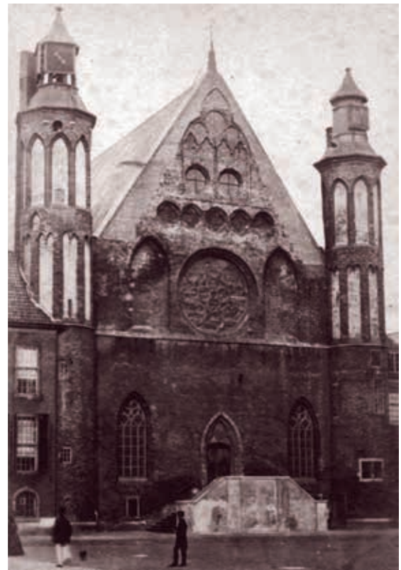
3B. The gable in 1865, following the replacement of the 1295 timber roof structure with a cast iron structure by government architect W.N. Rose in 1861. Because this new roof structure had a different pitch, the gable was adjusted by means of new masonry in a different brick that was fairly crudely toothed into the original medieval brickwork (The Hague City Archives)
