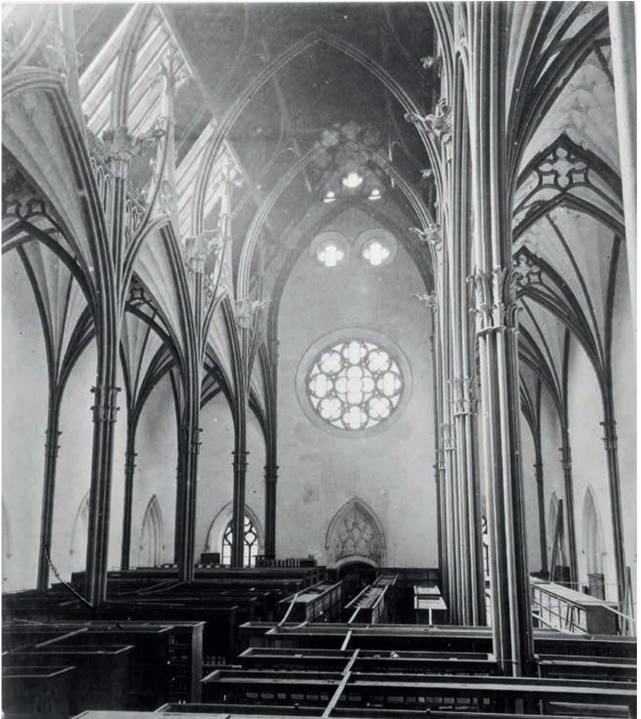
8. The Knights' Hall in use as archive room, with the cast iron roof from 1861 (Cultural Heritage Agency)
