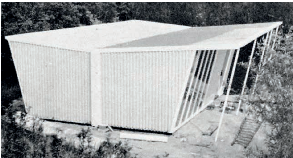
3. Wim Pijpers, plastic house, produced from 1962 by the firm Frits Bode Bouwplastic N.V. ( Bouw 18 [1963] 51)
