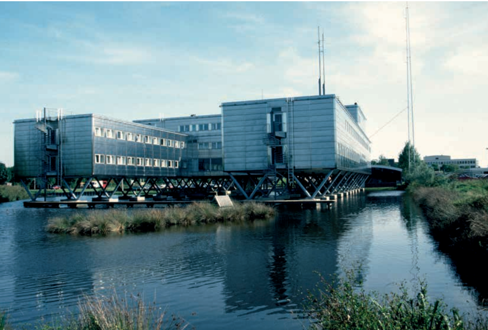
7. District Police Office in Groningen (1987) (photo Siem van 't Zet, Groninger Archieven)
