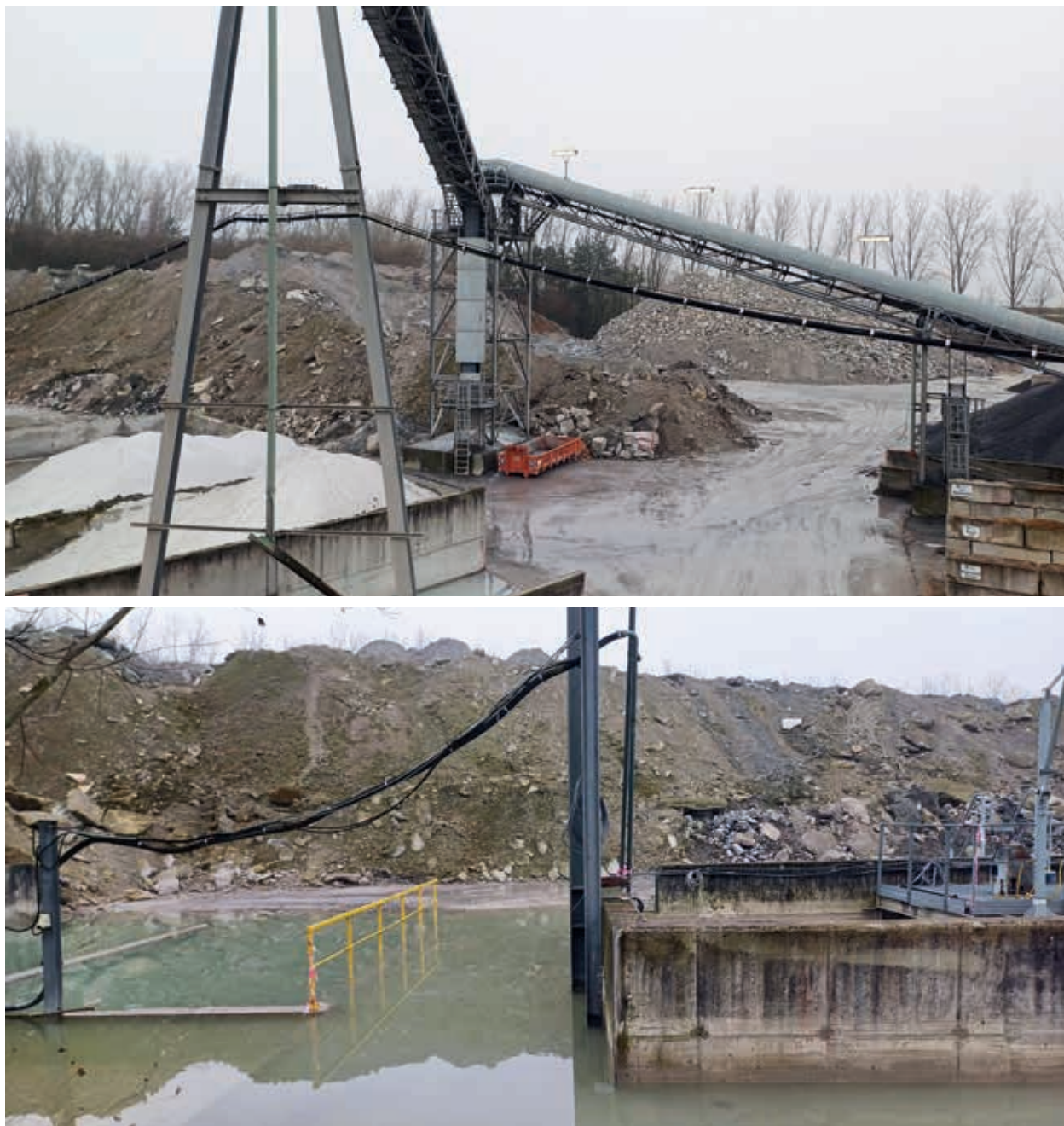
16. Large quantities of leftover cement and aggregate are flushed out when cleaning the mixing machine between different batches at the concrete plant in Sint-Pieters-Leeuw. Today, they are recovered in sedimentation basins, in compliance with environmental regulations. What previously happened to these leftovers, and with what environmental impact, remains unclear (Photo Tom Broes)
