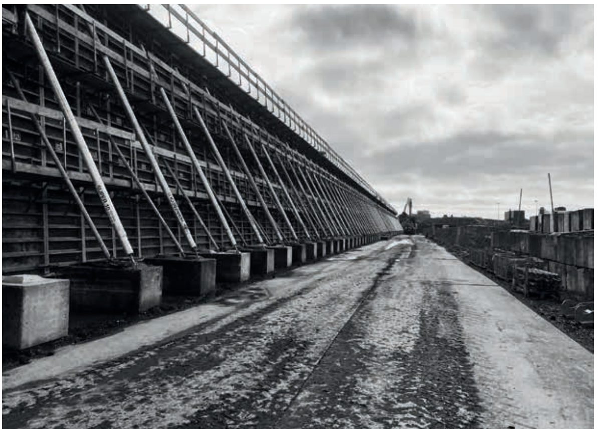
6 AND 7. Construction of an earth wall along the perimeter of a soil bank in Utrecht (photo C. Pradel)
